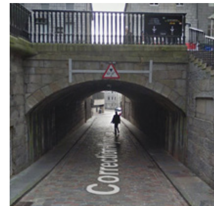
Correction Wynd underpass
