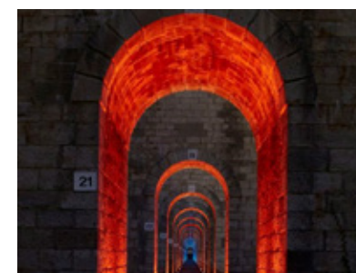
Project: Chaumont Viaduct, Chaumont, France Reference: www.iguzzini.fr
