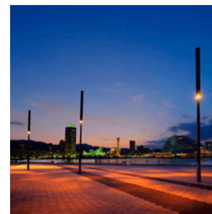
Solar powered luminaires
